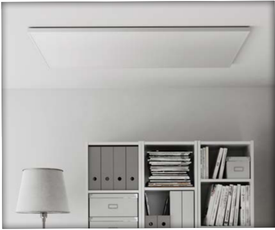
Ceiling mounted heating system
